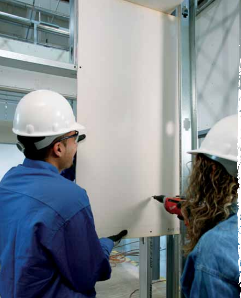
Figure 12 Top-down installation
