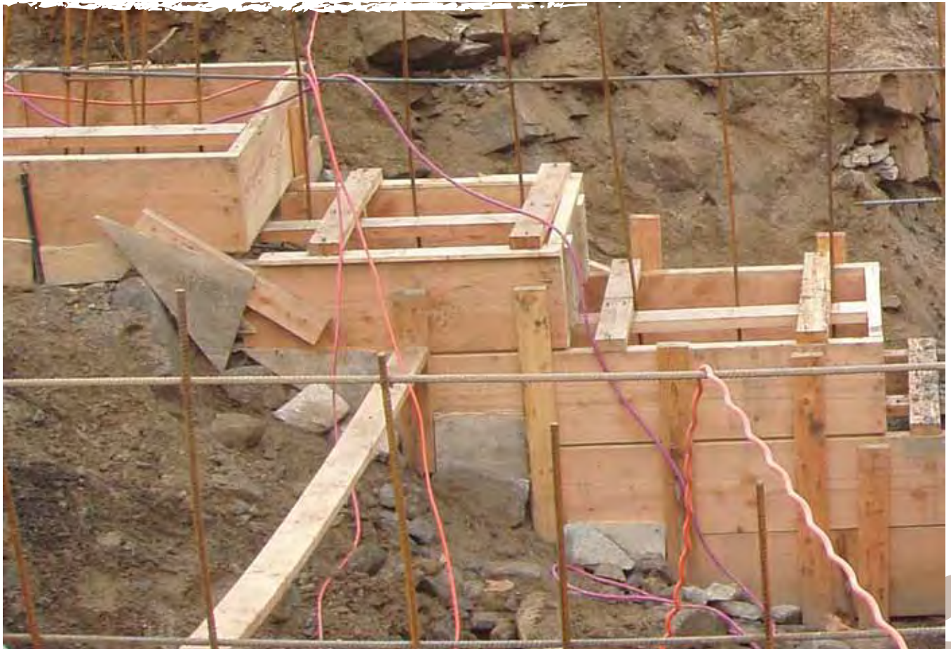
Figure 8 Stepped footing
