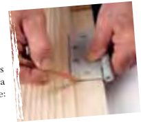
Figure 11 Drawing around the hinge
