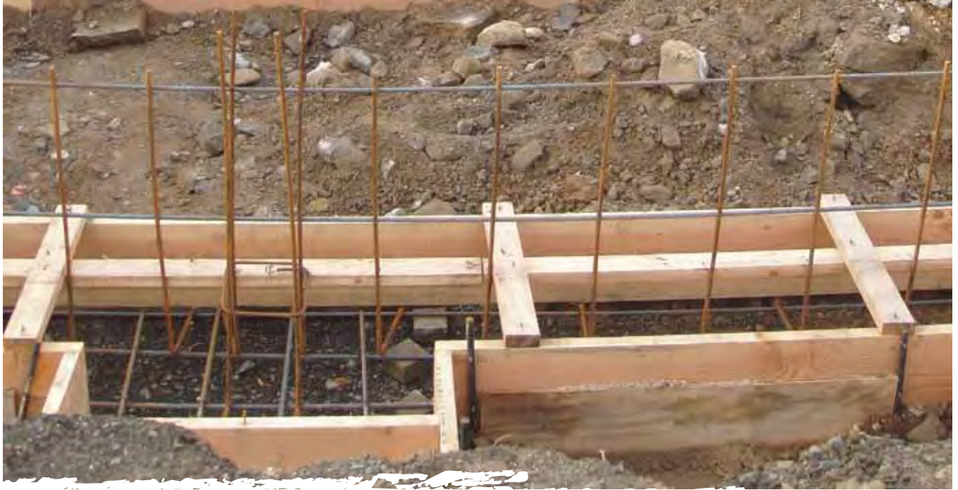
Figure 13 Steel reinforcing bar
