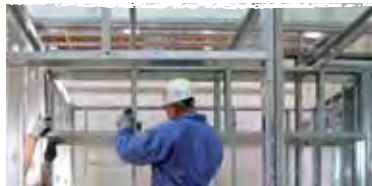
Figure 26 Fastening the horizontal studs
