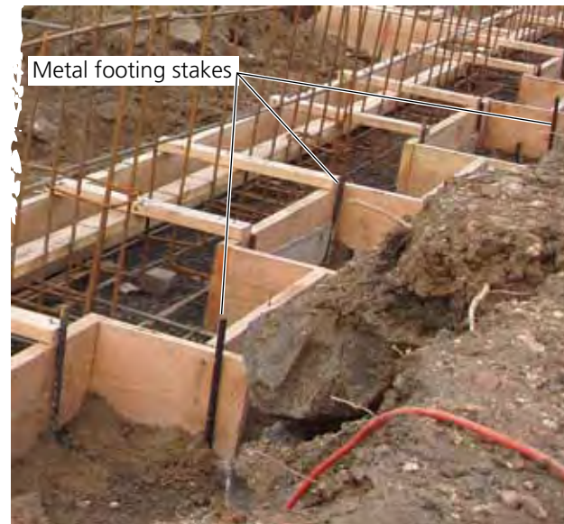
Figure 4 Metal footing stakes
