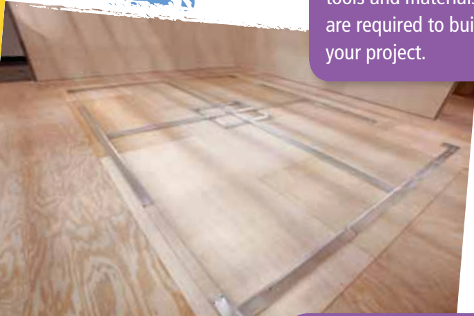
Figure 45 Perimeter bottom track installed
