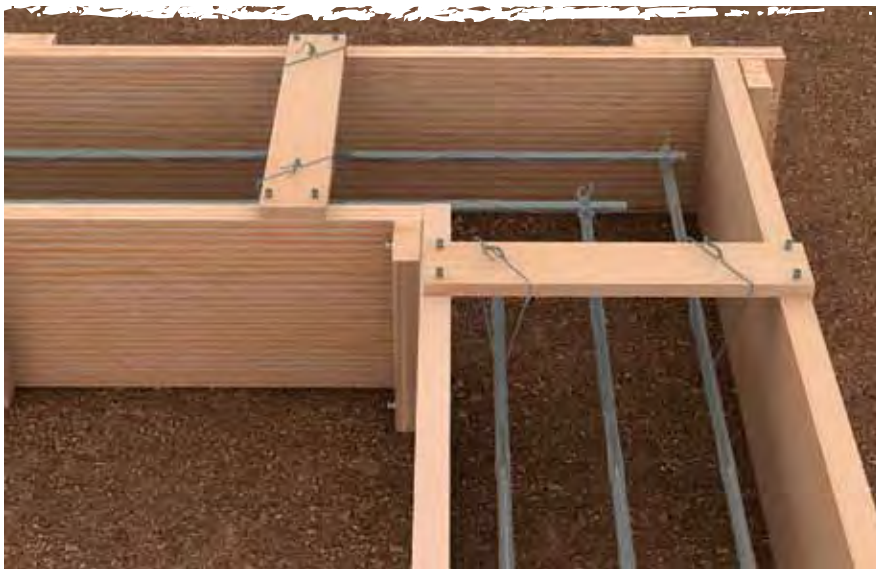
Figure 14 Reinforcing bar suspended by wires
