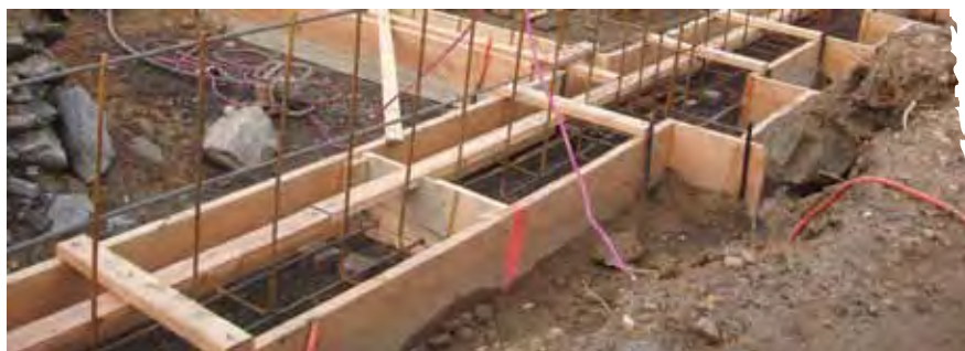
Figure 11 Footing forms in place
