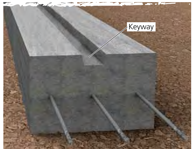
Figure 18 Keyway in the footer
