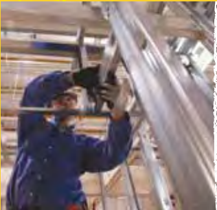
Figure 24 Installing the horizontal studs
