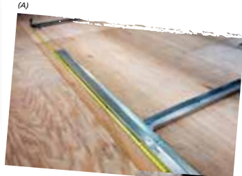
Figure 46 (A) Pulling the stud layout (B) Marking the stud layout
