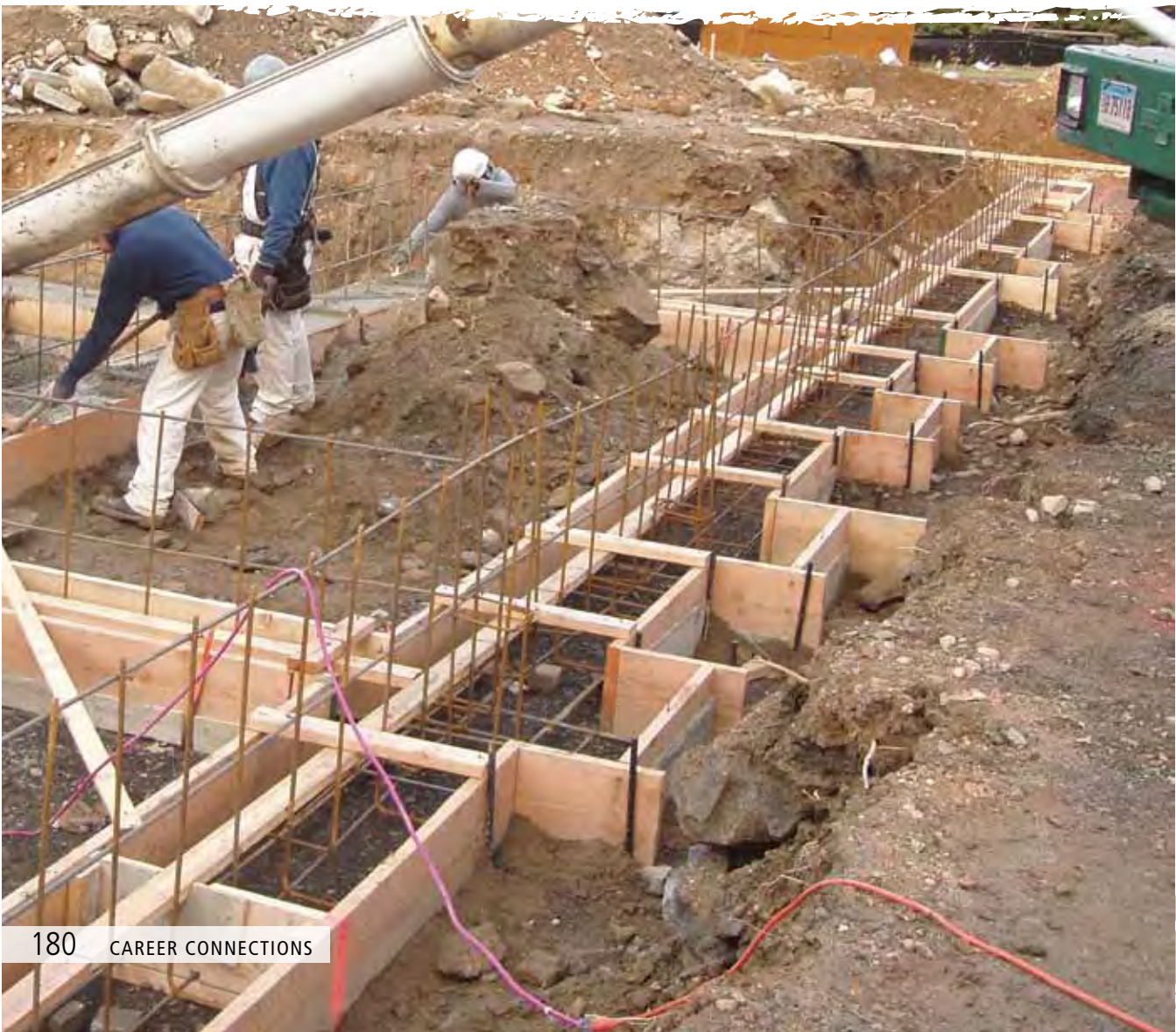
Figure 7 Continuous footing
