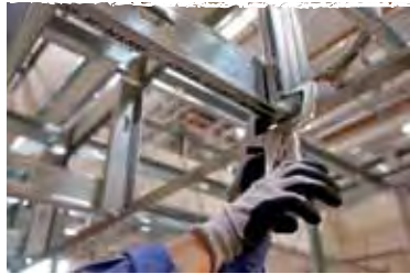
Figure 25 Clamping the horizontal studs to the wall angle
