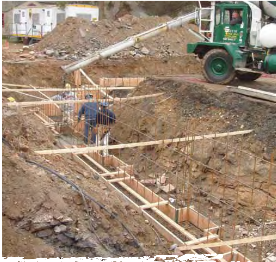
Figure 12 Footing forms being poured
