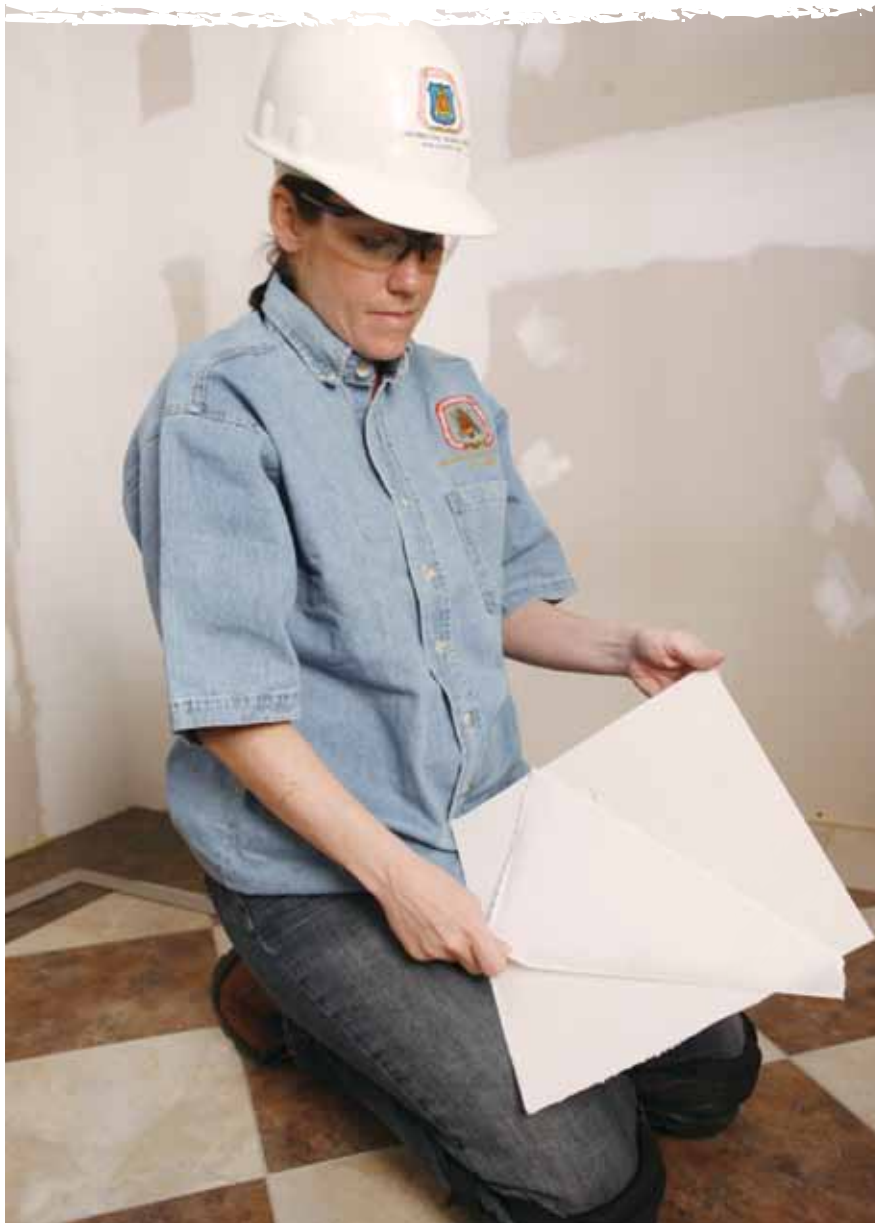
Figure 8 Removing backing from tile
