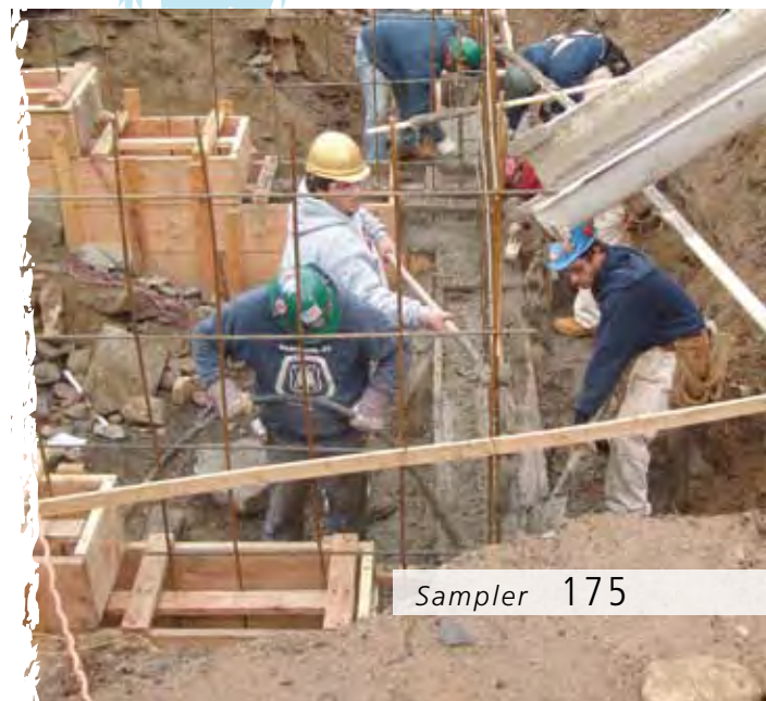
Figure 1 Placing concrete in forms
