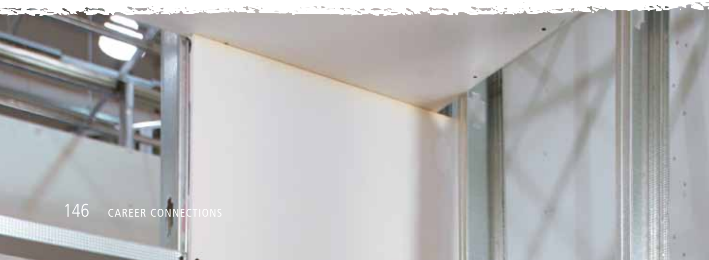
Figure 13 Sheet placed tight to the ceiling
