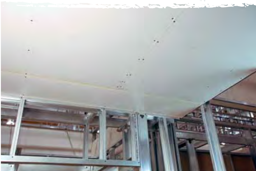
Figure 9 Completing the installation process
