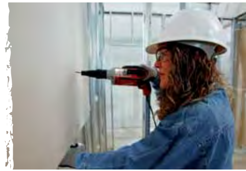
Figure 14 Placing screws in the sheet field
