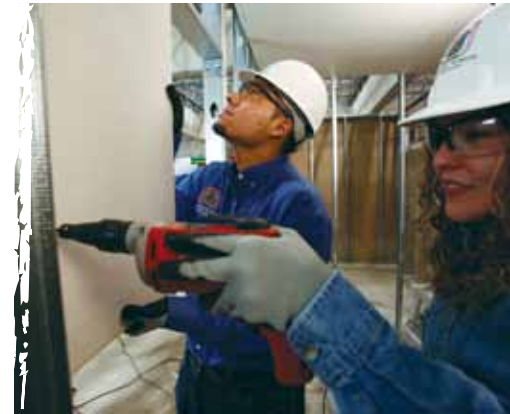
Figure 15 Fastening the perimeter
