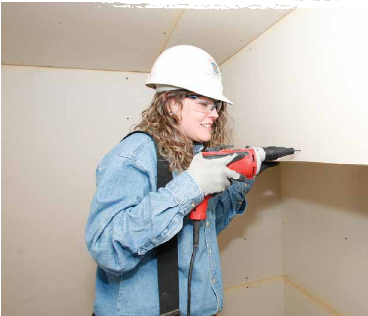
Figure 5 Correct screw attachment
