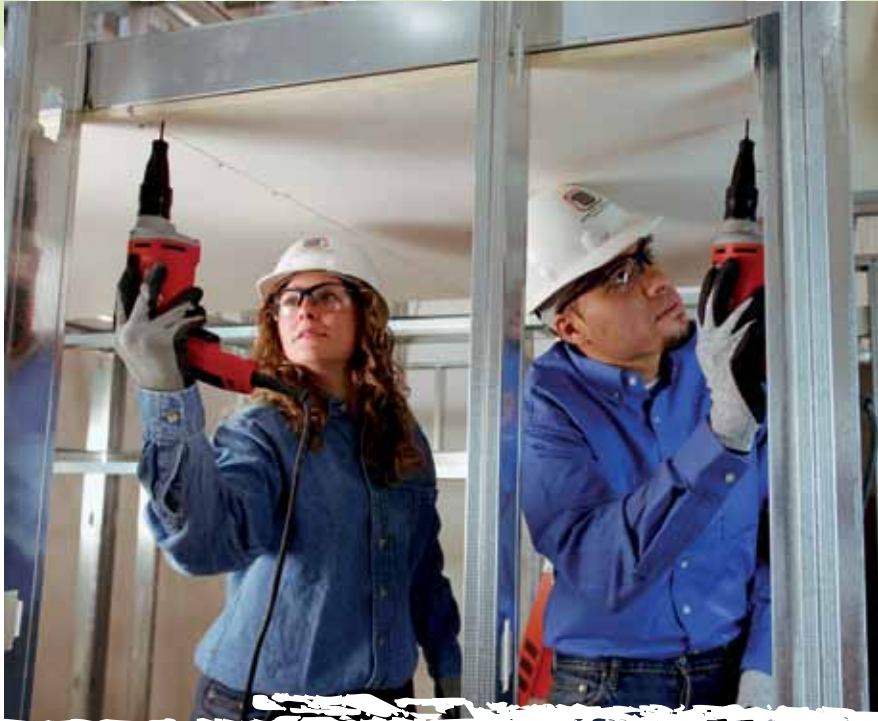
Figure 8 Placing screws in the field
